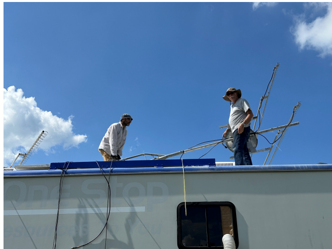
Assembling the microwave antenna array on the bus roof
