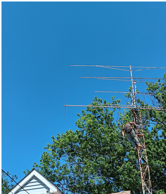
Doc's antennas being taken down.
